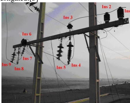
Figure 4. Online leakage current monitoring
